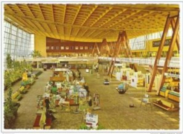
Brussels Airport has commenced renovation works on the roof of the Sky Hall, the former transit hall at the airport. It was a striking architectural choice in the fifties to have the roof rest on pillars in the middle of the space so that it seems to hover above the hall. The engineers of Brussels Airport Company have come up with their own out-of-the-box solution for the renovation so that the roof can continue to hover and the iconic look of the Sky Hall is retained.
